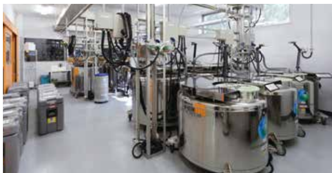
▲ Liquid nitrogen tanks
